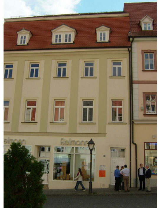
CCG's new office in the historic building faces the statue of the reformer Dr. Martin Luther in the market square. Luther's birthplace, a memorial since 1693, is the oldest museum in the German-speaking area.
