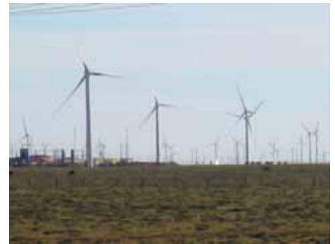
Up to 1,000 towers can occupy one wind farm.
